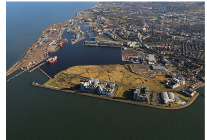
Aerial view of reclaimed land
